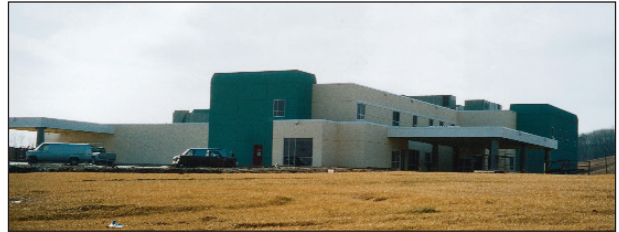
New Mountainside Medical Center
