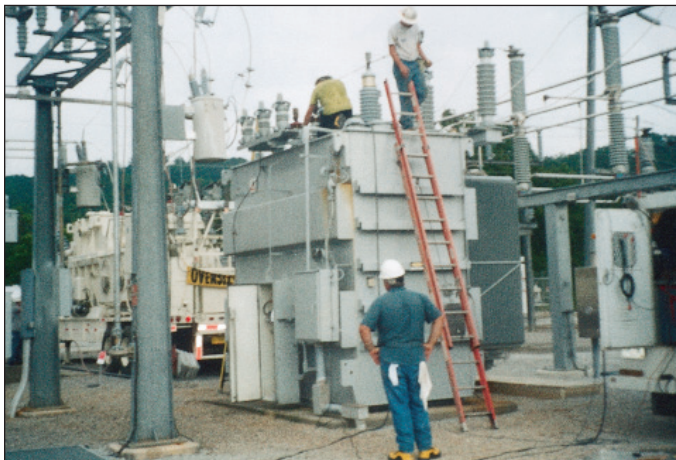
Crews replace a transformer that failed due to lightning damage.
