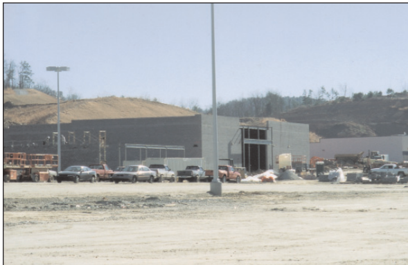
New Goody's under construction.
