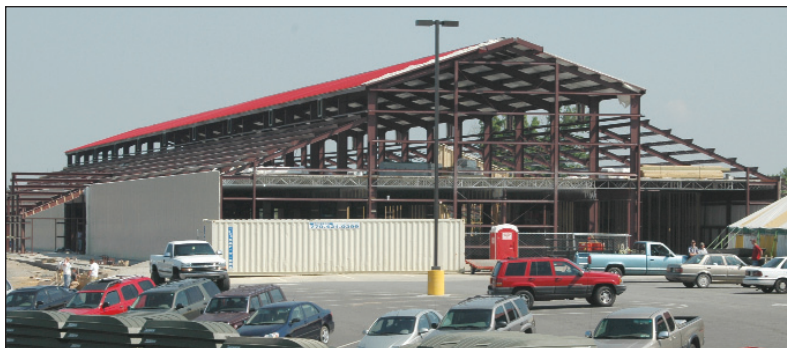
Bargain Barn reconstruction almost complete.
